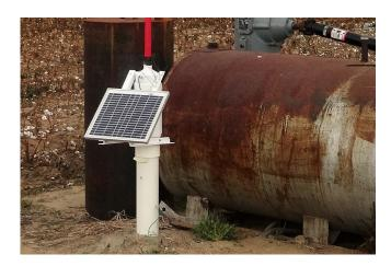
The DP1 provides monitoring and control for pumps that help prevent pump failure and reduce downtime.
